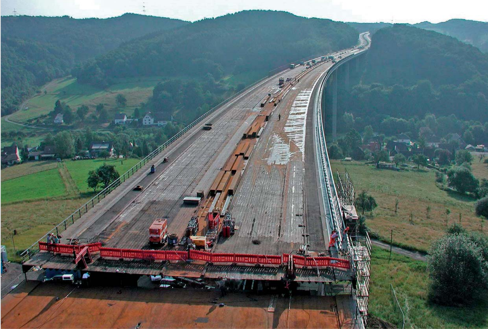
Wiehltal highway bridge, Germany.
